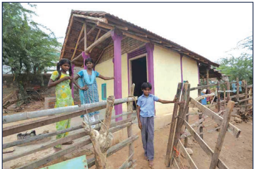
Decent housing, easy to construct, for low-income families in Bhuj, Kachchh
